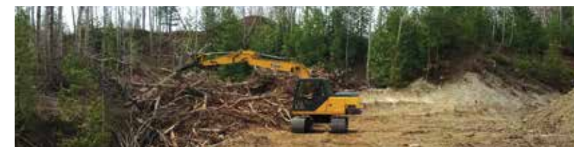
REINFORCING SIDE SLOPES WITH HARVESTED WOODY DEBRIS. NO MATERIAL GOES WASTED!
