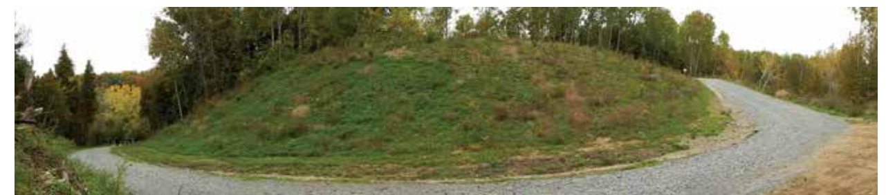
OCTOBER 2015 THE GRASSES HAVE GERMINATED AND THE ROAD IS OPEN TO THE PUBLIC.
