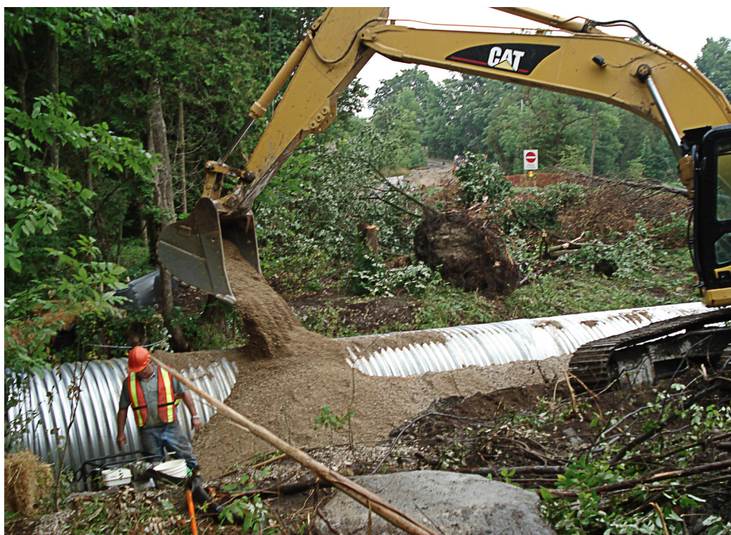
Culvert installation in Town of Chesley.
