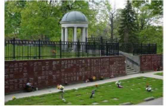
COLUMBARIUM RETAINING WALL
