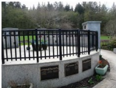
MEMORIAL PLAQUES AT RETAINING WALL
