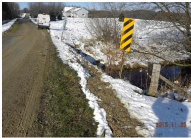
Drain 86 Structure L located on the 3<sup>rd</sup> Line between Bride Road and School Road 7 requires re-construction within 25 years. As shown in the picture there are no guiderails at
