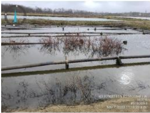
Figure 6c: Filter Cell 2 (facing north)
