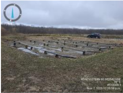
Figure 6a: Filter Cell 3 (facing north)
