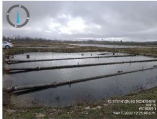
Figure 6b: Filter Cell 1 (facing north)
