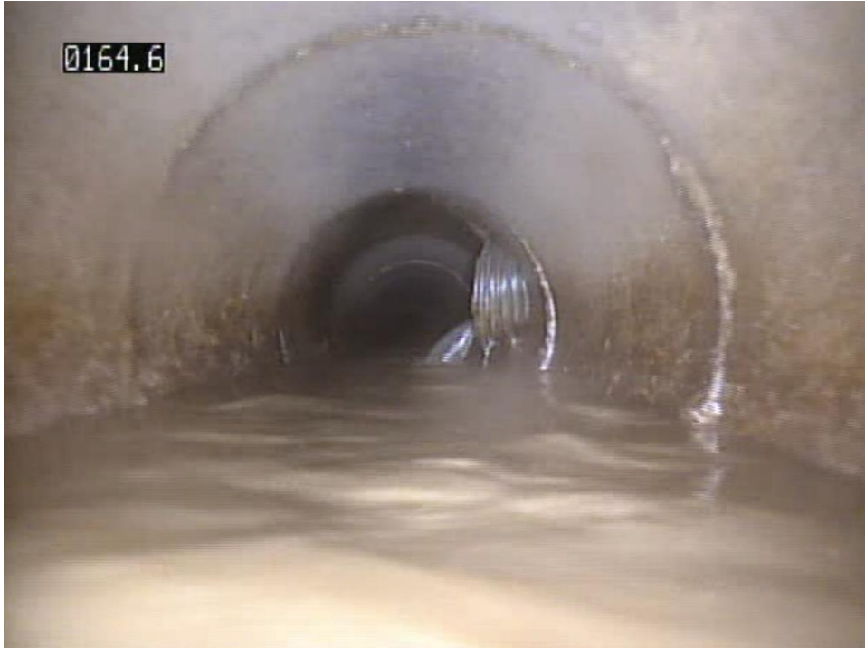
Figure 5 – Branch C connection to Main Drain
