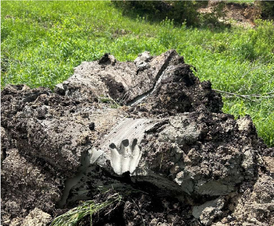
Figure 2 – Unstable clayey soil with the low-lying lands on Lot 7, Concession 8
