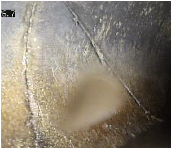
Figure 4 – Tile cracks
