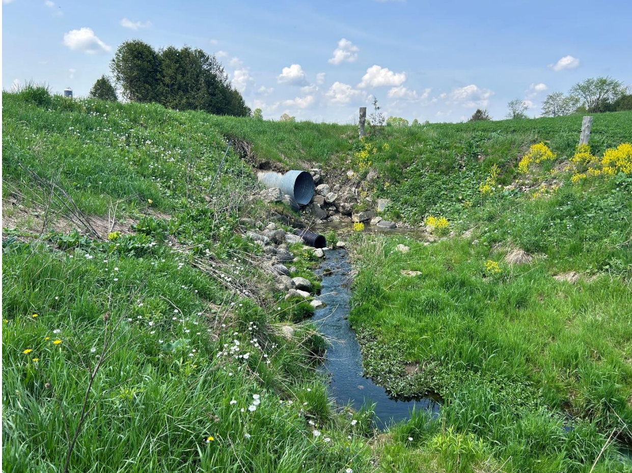
Figure 2 – Open portion of Minto Drain No. 14 just north of 8 th Line
