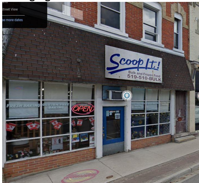
Existing Sign and Storefront
