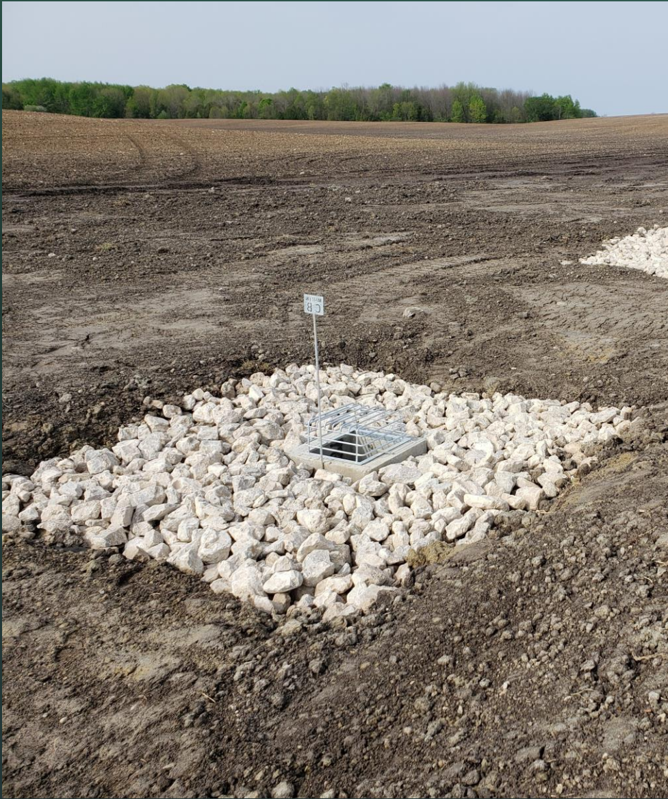
Catchbasin Installation
