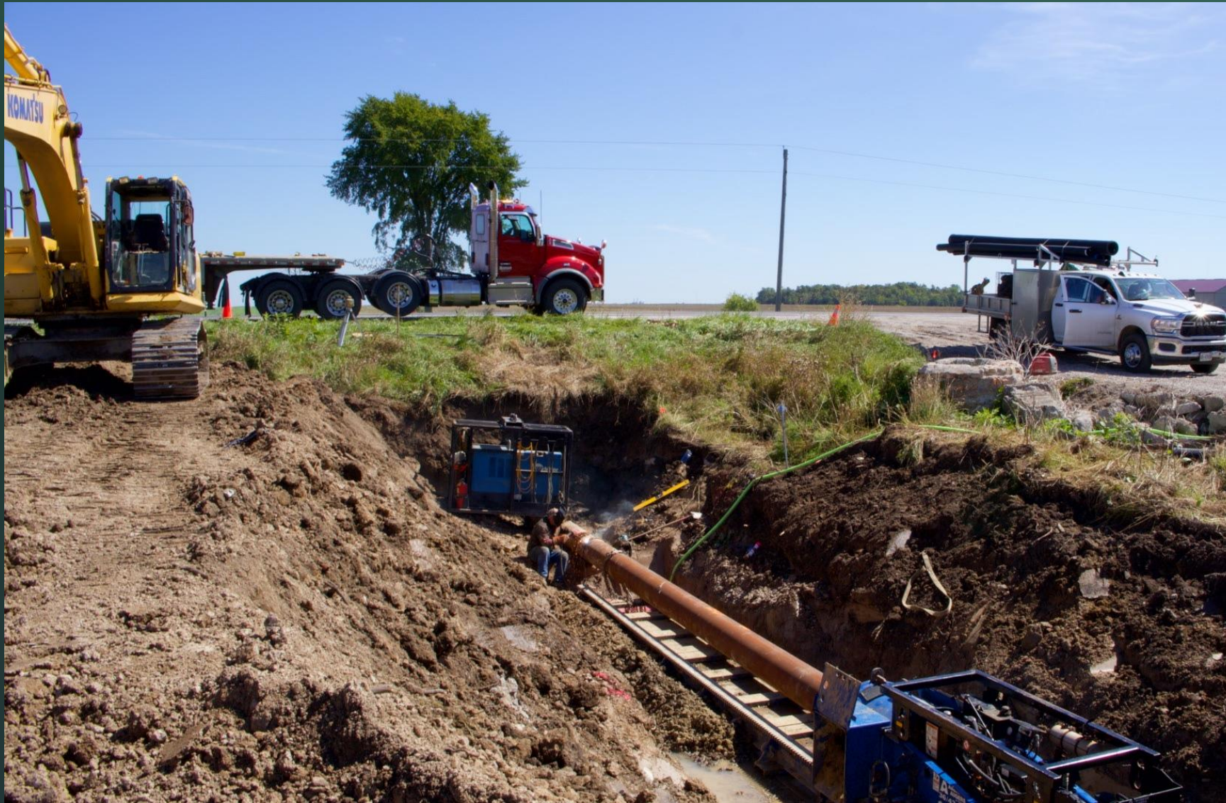
Smooth Wall Steel Casing Installation (Jack and Bore Method)
