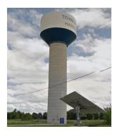
b) The Harriston System (Class II) serves about 2,108 permanent residents and 800 households. It contains three drilled bedrock wells, three wellhouses, an elevated 1915 m³ storage tank and a distribution network of 100 mm to 250 mm mains. About 77 fire hydrants are available for fire protection. There are 830 active water meters. Peak water consumption was 388,458 m³ in 2009, and the lowest consumption in 2016 was 287,099 m³, a 26% reduction. Average consumption is 354,861 m³ per year since
