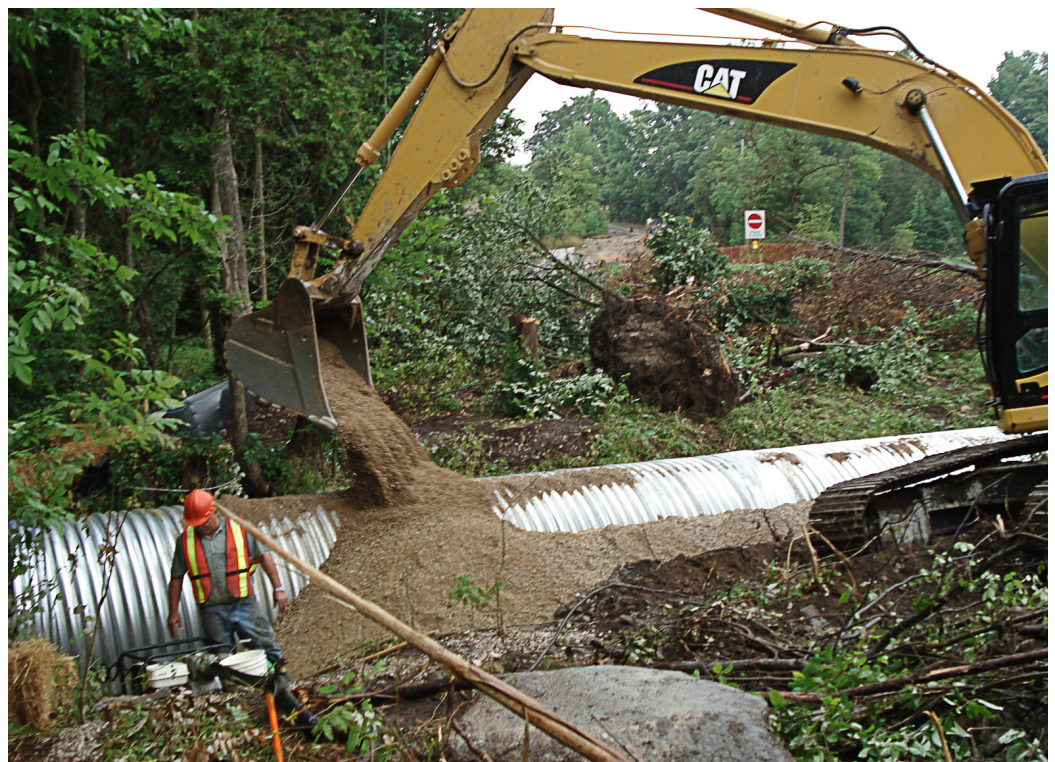
Culvert installation in Town of Chesley.
