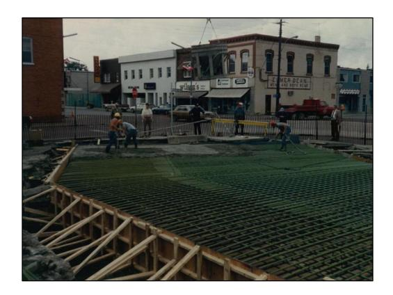
Buildings over the conduit were removed and the conduit was reconstructed to handle the 100 year flood. This meant that the flood risk went from a 15% chance of it happening in any year to a 1% chance.
